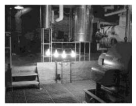
The world's first usable amount of electricity from nuclear energy was produced by Experimental Breeder Reactor 1 in Southeastern Idaho and used to light these four light bulbs on December 21, 1951.
