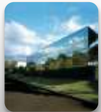
Maui High Performance Computing Center DSRC
