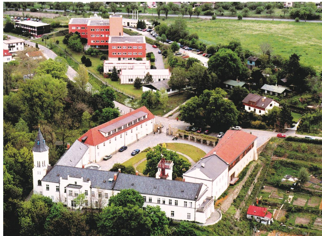
CHMI headquarters at Prague
