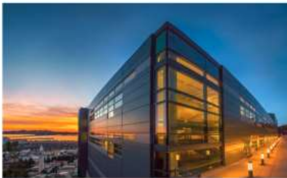
Photo Credit: LBNL. Shyh Wang Hall, home of NERSC, the Lab's high performance computing center.
